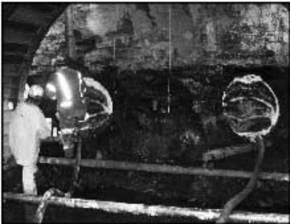
Back filling Auger holes
