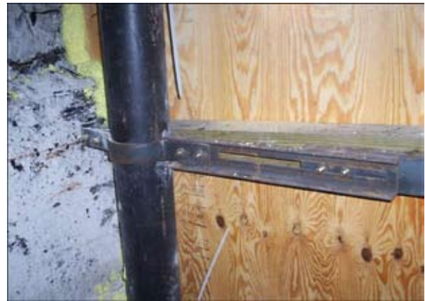
Plywood secured to supports
