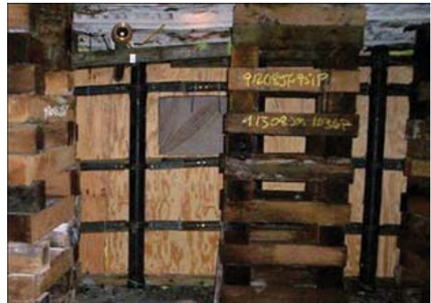
Completed Plug Seal
