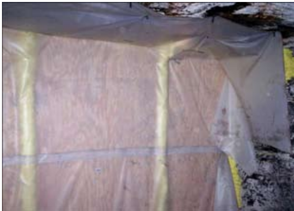
Formwall sealed with foam sealant and plastic prior to Stratacrete pumping
