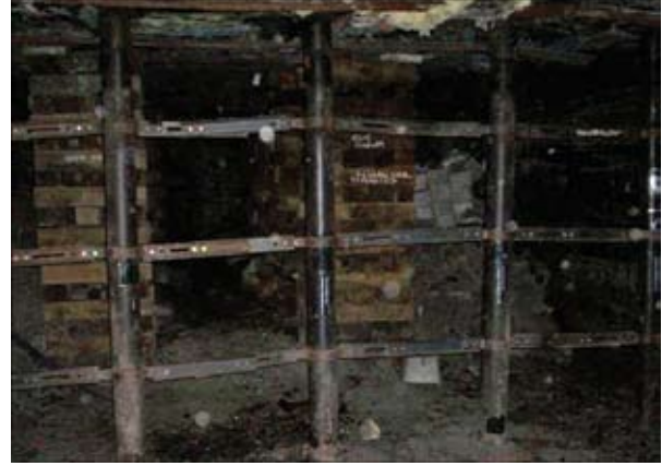
Formwalls constructed using prestressed Rocrops™ and support clamps*
