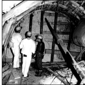
Ventilation Stopping built using Rocsil
