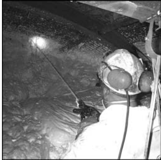
Rapid spray-on application
