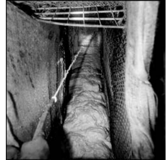
Maingate Stopping - France
