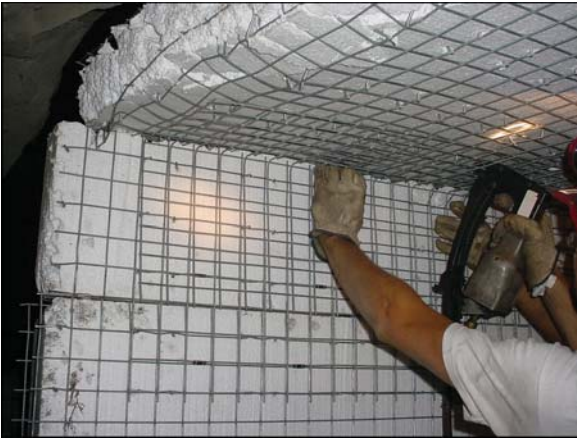
Constructing overcast
