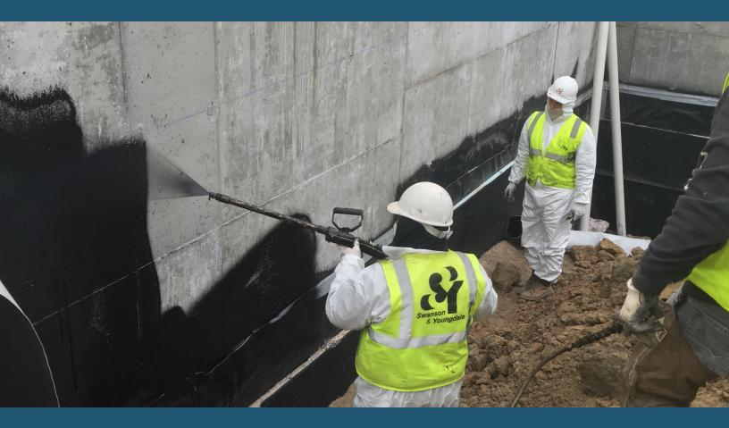
GEL-TECH SYSTEMS is a composite waterproofing system that incorporates a cold fluid applied GTS Polymer Rubber Gel with a high performance GTM Protection Sheet. The combination of a non-curing, self-healing, Polymer Rubber Gel, with a durable puncture resistant protection sheet, makes GEL-TECH the ultimate waterproofing solution for above grade, below grade and blind side applications in mining and tunneling.
