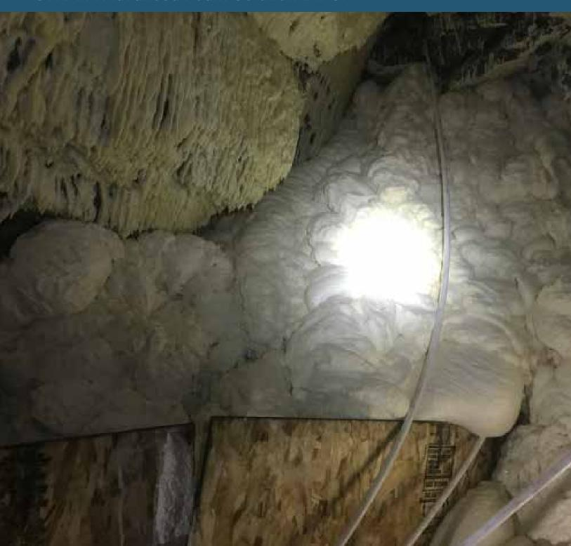
Strata AFS is a hydrophobic polyurethane, designed to be injected into rock fissures, gravel layers, joints, cracks and voids to fill voids and consolidate strata. It is ideal for controlling and diverting water, including high volumes of gushing water.
