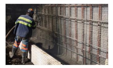
The Strata 3D Spray panels are two layers of galvanized steel-mesh on either side of an expanded polystyrene core. Designed and welded for rigid strength and flexibility, the 3D panels are easily cut to size and fastened together for a variety of construction applications. Sprayed with a concrete coating, the final structure is strong, air-tight and fire resistant. The polystyrene core maximizes flexion to absorb overpressure from blasting.
